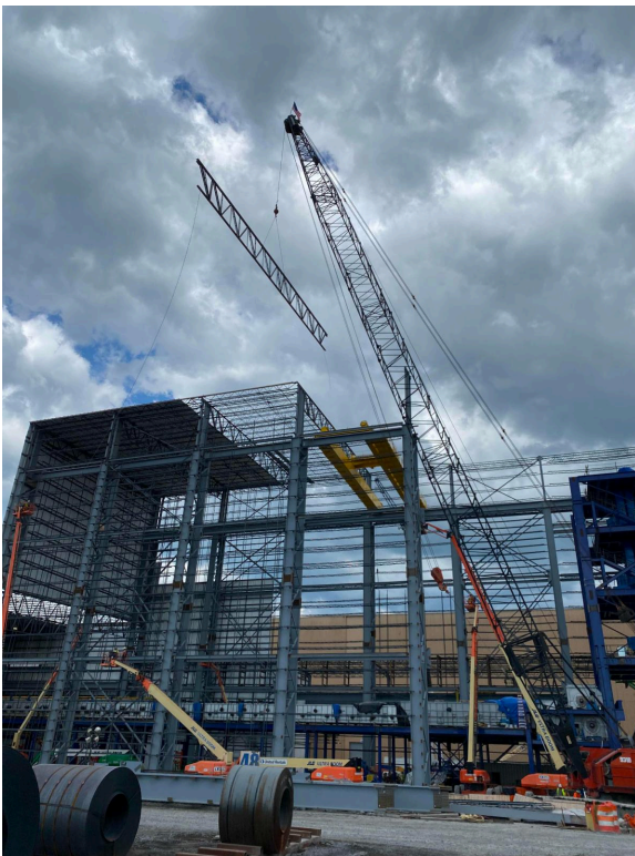
Southern Industrial Contractors recently performed the work shown in the photos above which included 7,600 tons of structural steel with eave heights of 135 feet, numerous overhead crane installation, and 700,000 SF of wall sheeting, roof cladding, and 6-inch batt insulation.
